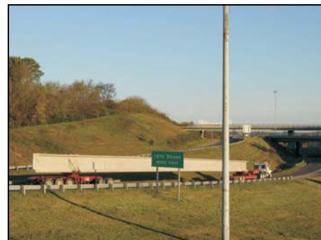
For this Birmingham bridge reconstruction, Sherman provided the longest prestressed girders ever used in Alabama.
